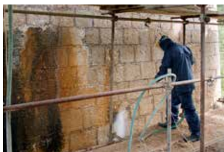
Cleaning building scaffolding
